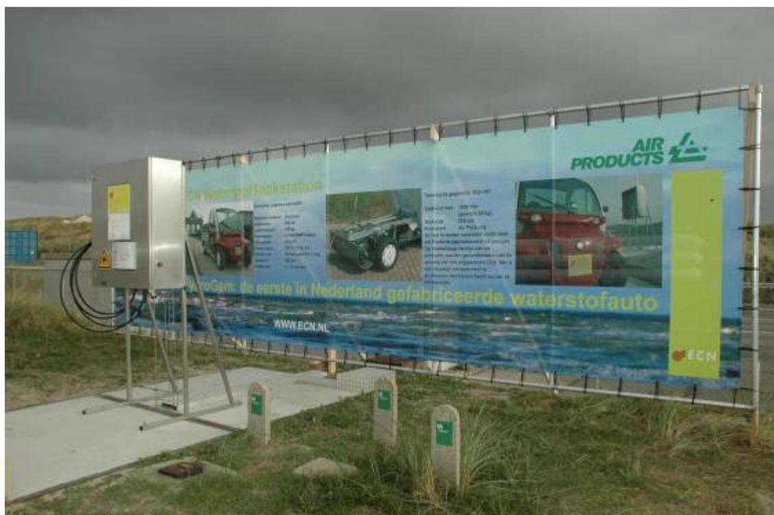
Figure 9: Photo of the 200 bar hydrogen filling station delivered by Air Products
